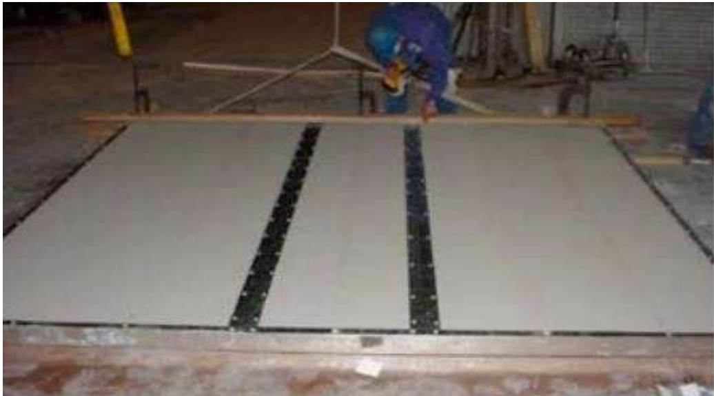
JOINTING SHEETS FOR INSTALLATION
